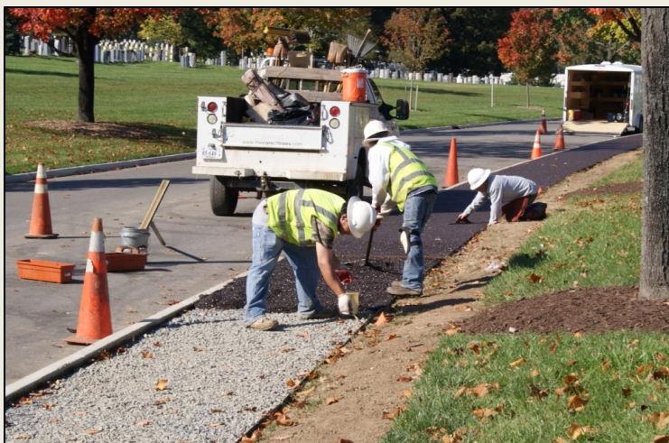
Contractors spread the softened rubberized material evenly over gravel to form the new sidewalks along Eisenhower Drive. Photo by Melissa Bohan
